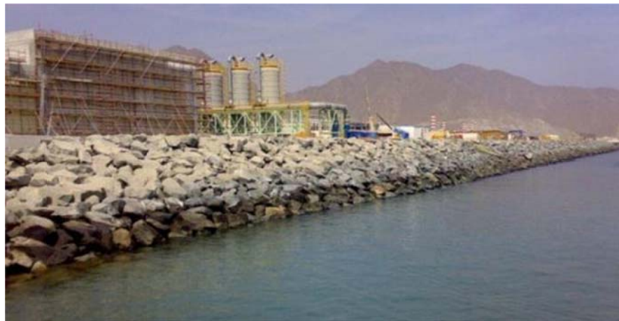
Fig. 4: Photograph shows the Existing Seawall
